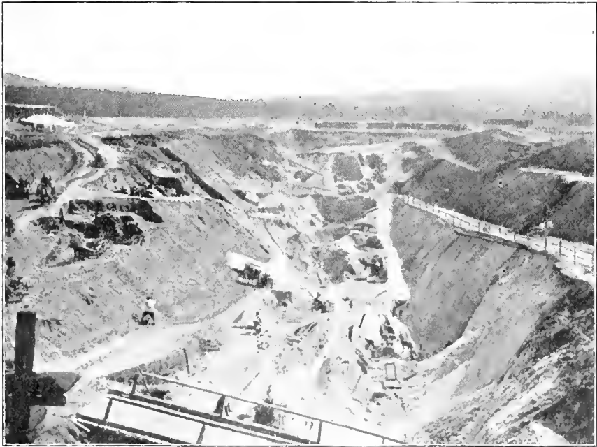
SOUTH END OF THE OPEN-CUT WORKINGS AT THE TISSOFF MINE.
